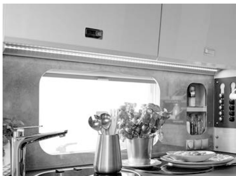
Fig. 60: LED light rail (typical)
