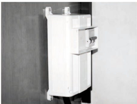
Fig. 57: Ground fault circuit interrupter (GFCI)
