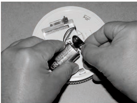
Fig. 162: Replacing the block battery
