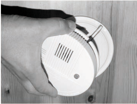
Fig. 161: Removing the housing
