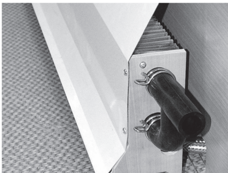
Fig. 91: Convector with thermally conductive panel
