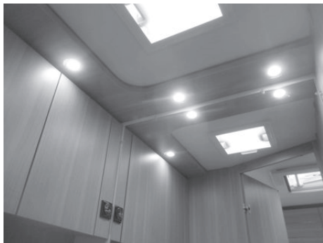
Fig. 66: Bathroom lighting, example
