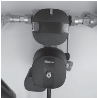
Fig. 78: Gas supply (with Eis-Ex and remote control)
