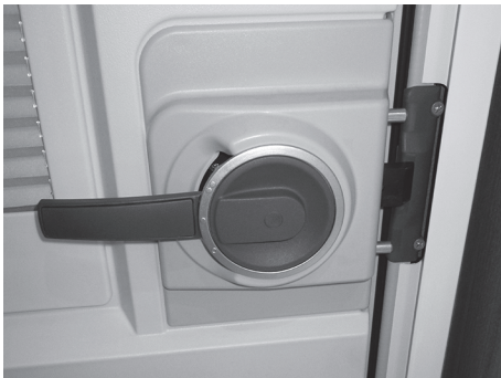
Fig. 15: Closed but unsecured door lock
